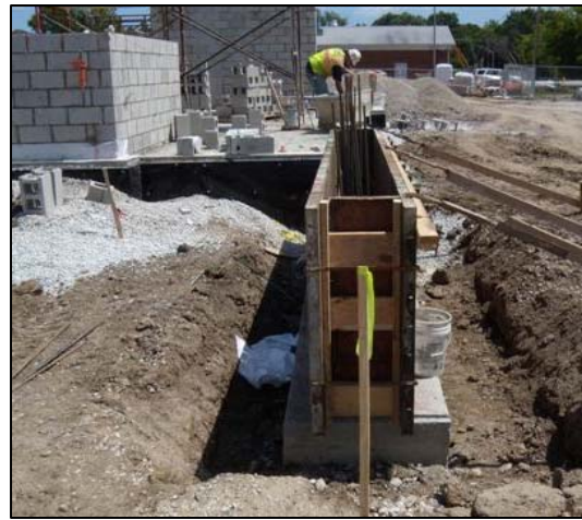
Monument sign work
