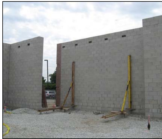
Interior block work
