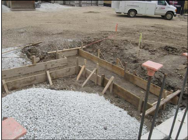
Framing footings for patio
