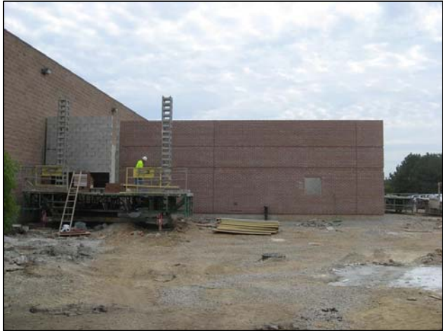
Block/brick work at the EOC (looking at west wall)
