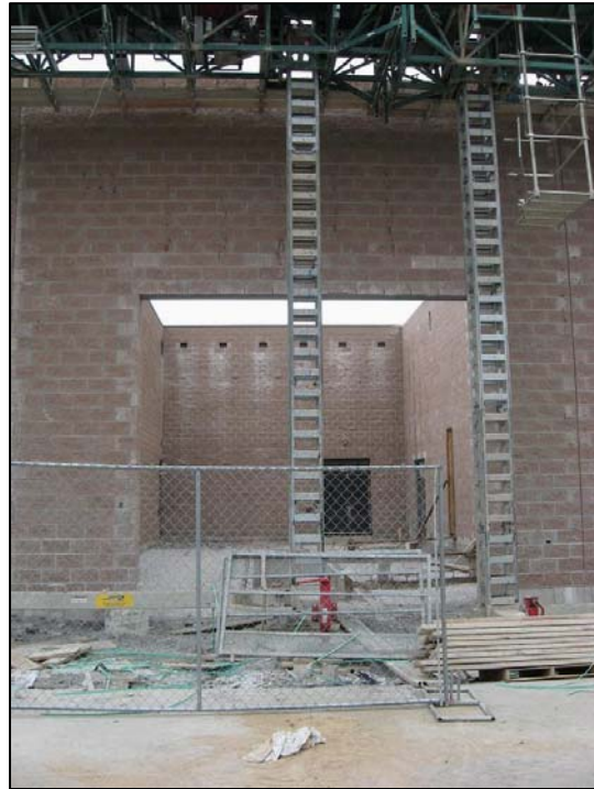
Looking into the new spray booth
