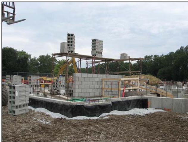
First floor block work
