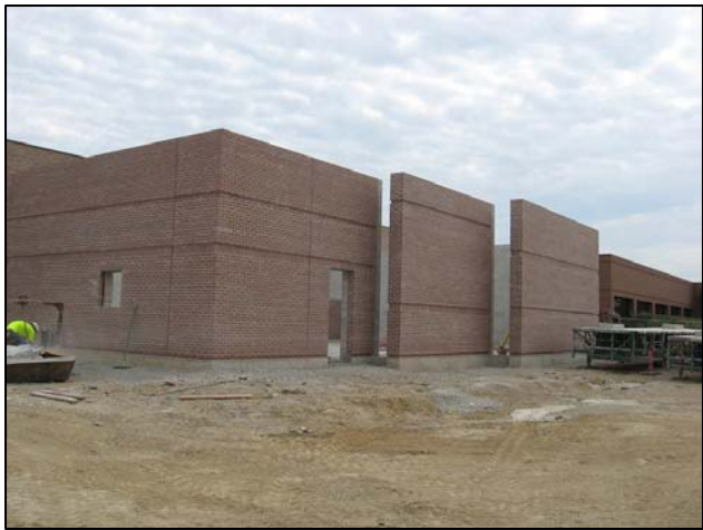
Completed brick work on south wall
