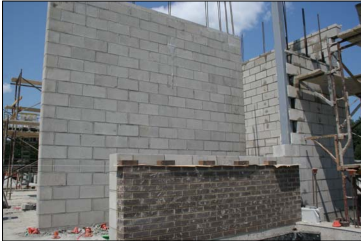
Block and brick work on the front stairwell
