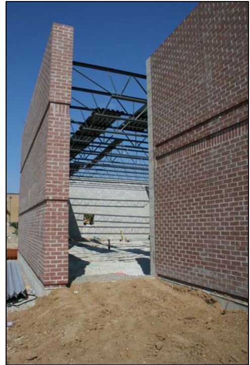
Steel work at front of EOC
