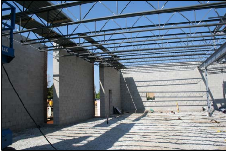
Steel roof structure
