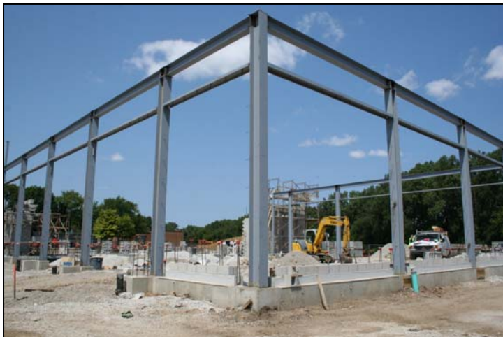
Steel work on the apparatus floor
