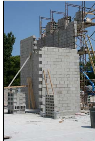
Masonry on the rear stairwell
