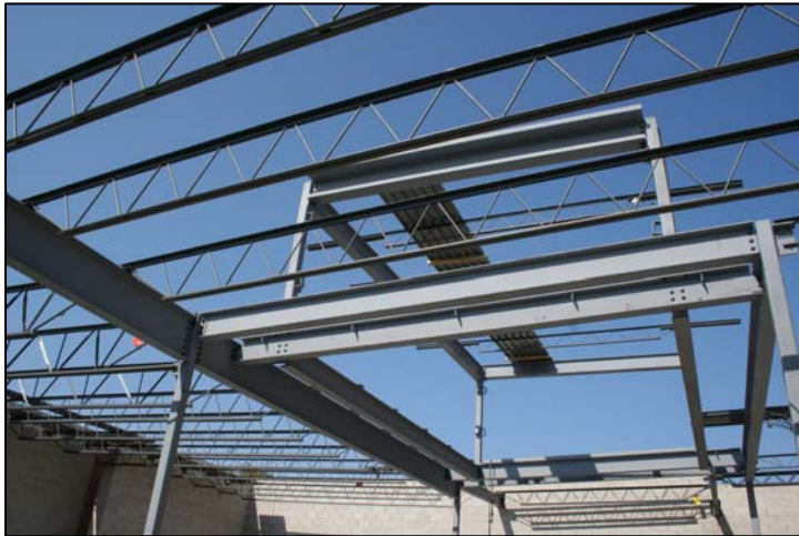
Steel frame work for clerestory windows in Command Room
