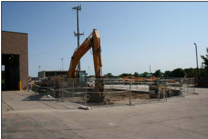
Prep work for new wash bay
