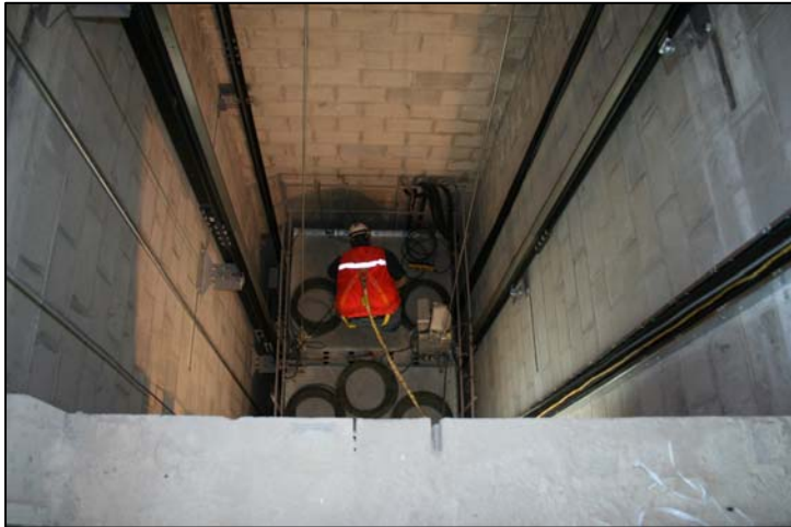
Working on installing the elevator
