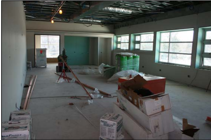
Second floor training room
