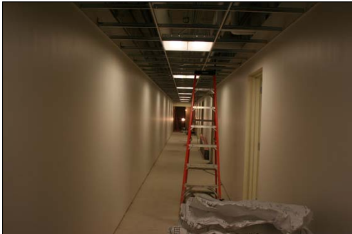
Drywall & ceiling grid progress in the basement
