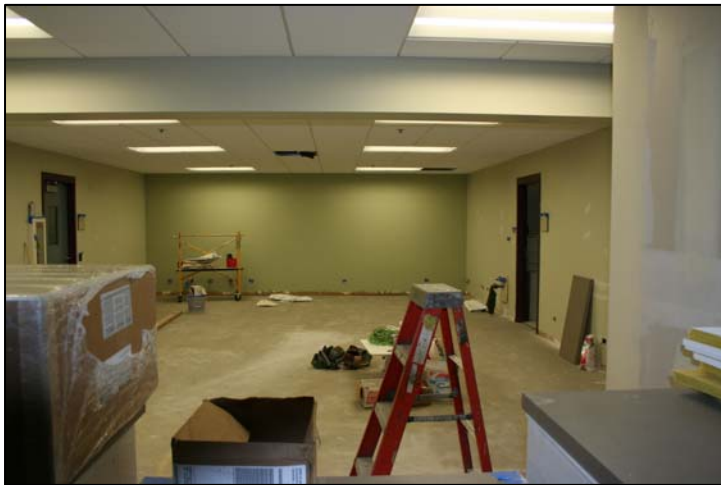
Remodeling work in the lobby and front office space
