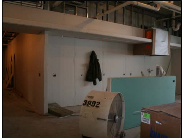
Drywall progress in the kitchen
