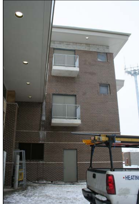
Railings on the training tower
